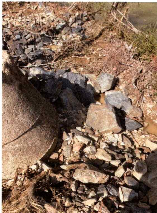
Manhole 1741 Before Cleanup
