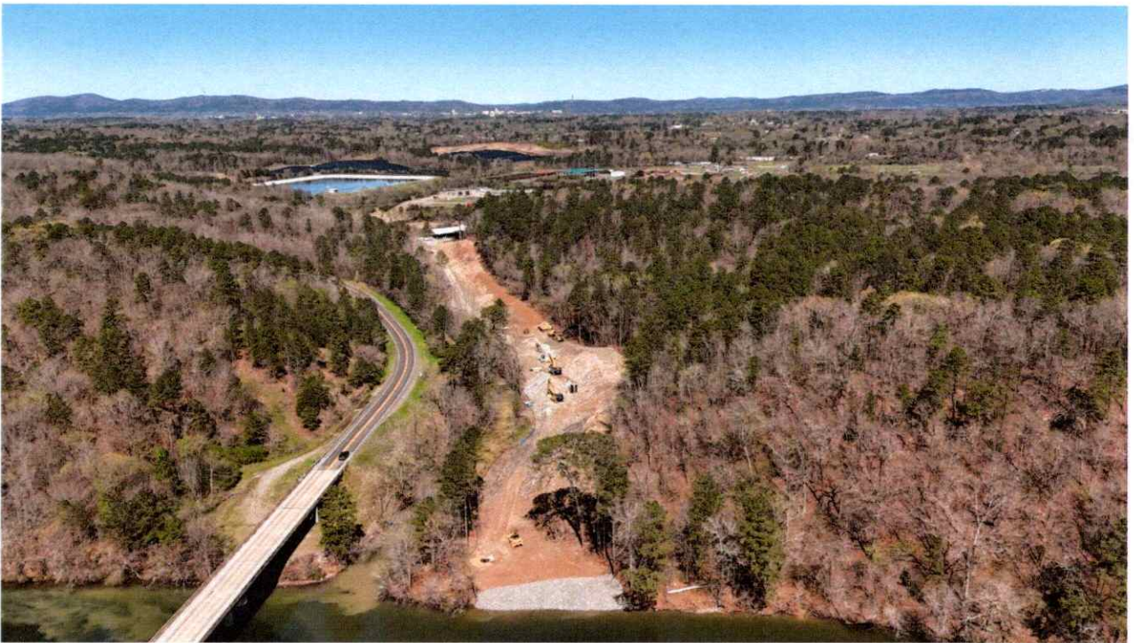
Davidson Drive WWTP Outfall Construction
