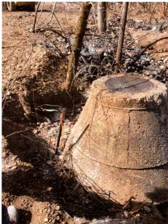
Manhole 1741 After Cleanup –
