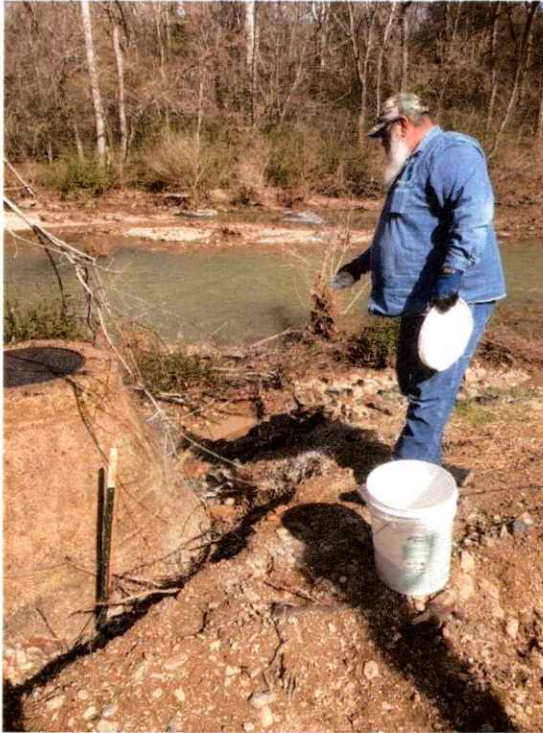
Manhole 1741 During Cleanup
