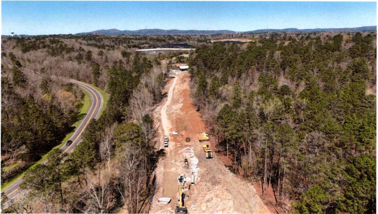
Davidson Drive WWTP Outfall Construction
