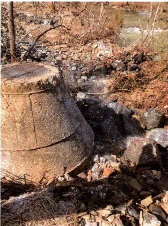
Manhole 1741 After Cleanup
