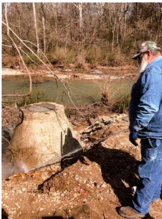
Manhole 1741 During Cleanup
