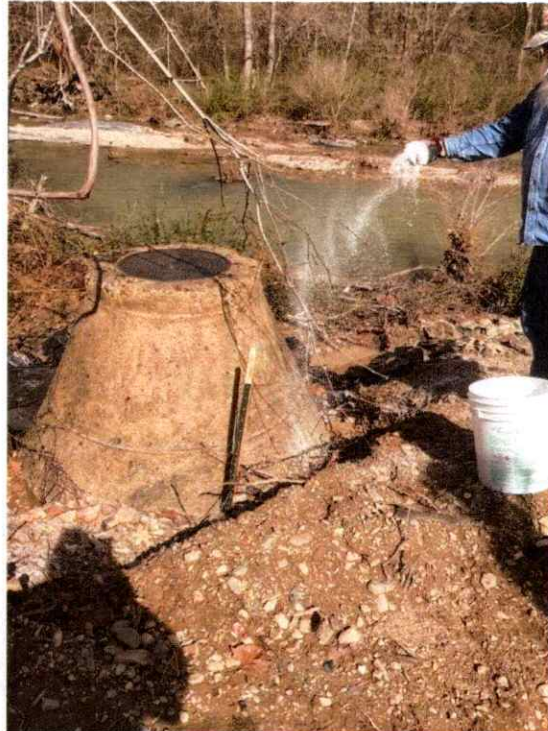
Manhole 1741 During Cleanup
