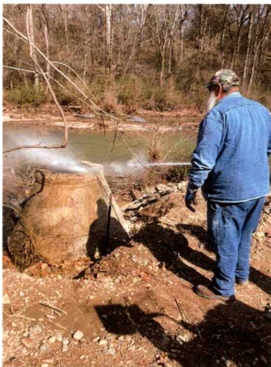
Manhole 1741 During Cleanup
